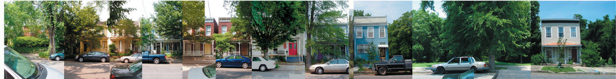
2. BROAD STREET ELEVATION LOOKING NORTH
