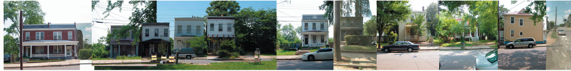
1. BROAD STREET ELEVATION LOOKING SOUTH
