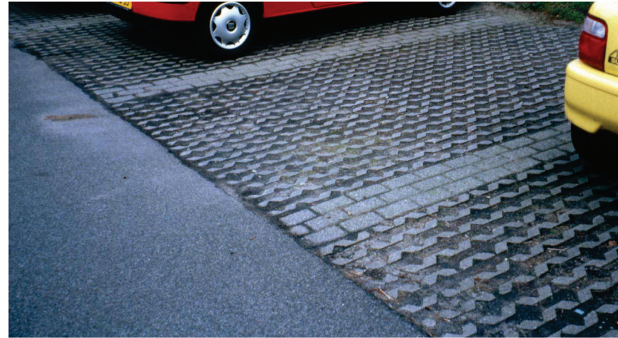
3 Porous Paving: Parking Spaces
