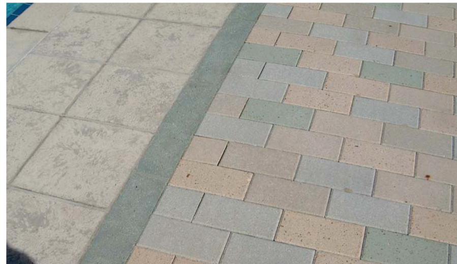
4 Porous Paving: Pavers
