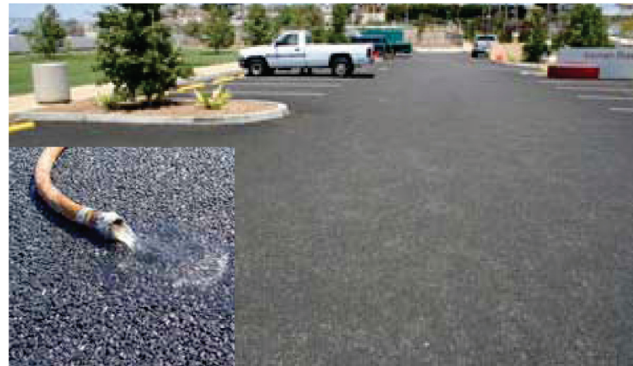
5 Porous Paving Concrete
