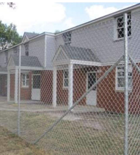
Creighton Court is lined with construction fencing during the upgrades.
