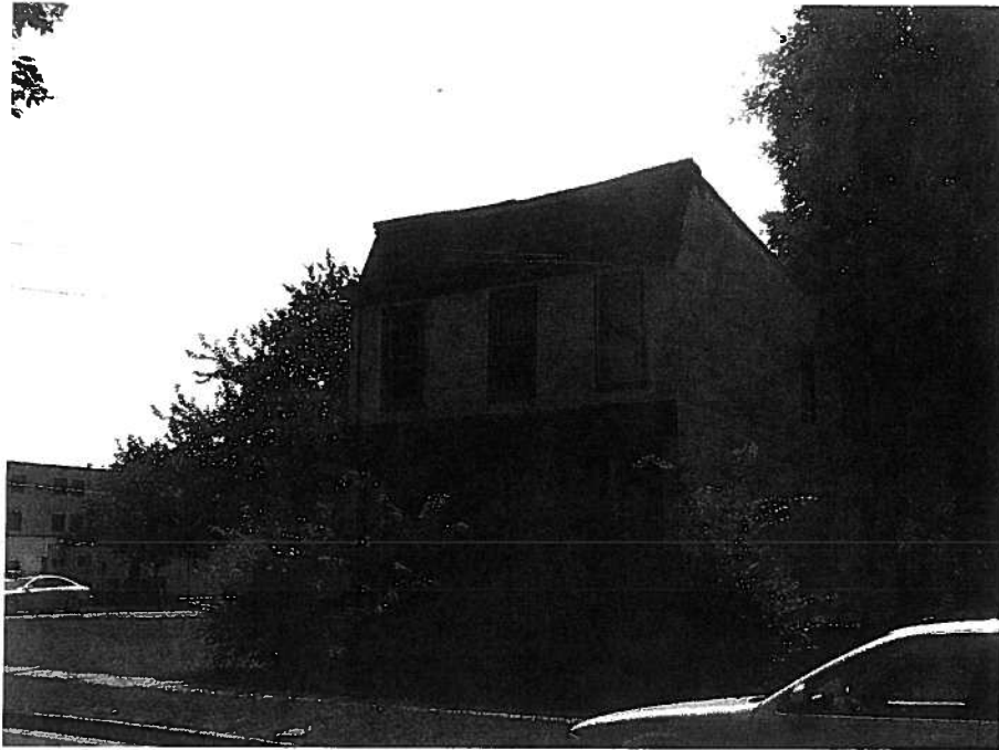
View of west and south elevations from the west (taken from 27 th Street)
