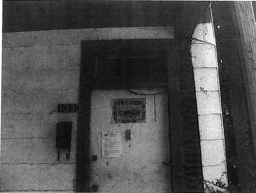
Detail of east elevation
