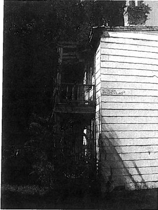
View of north and west elevations from the north (taken from the side yard)
