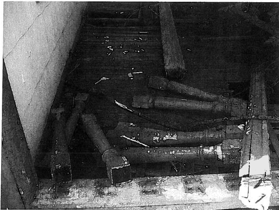
Detail of east elevation
