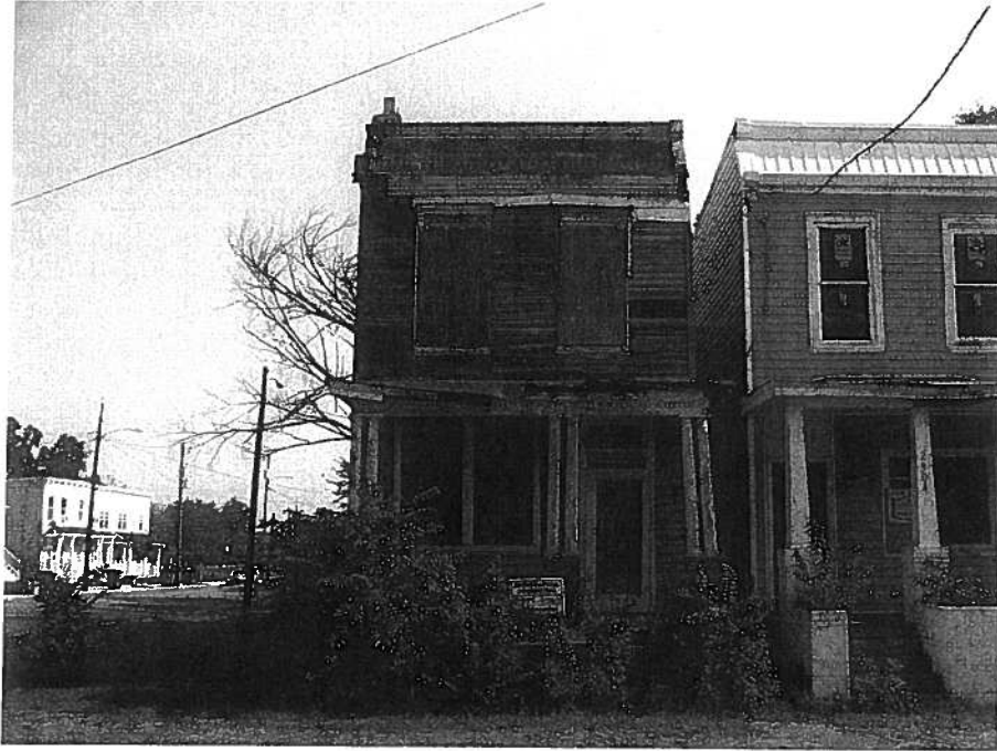
View of south elevation from the south (taken from Leigh Street)
