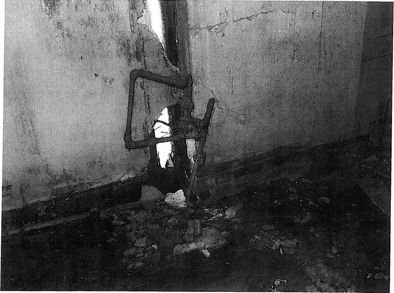
Detail of second floor interior
