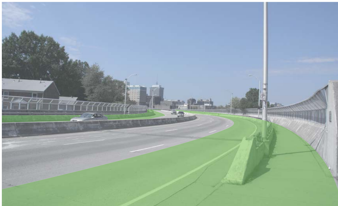
View of existing bridge, looking west - green overlay marks the zones for improvements
