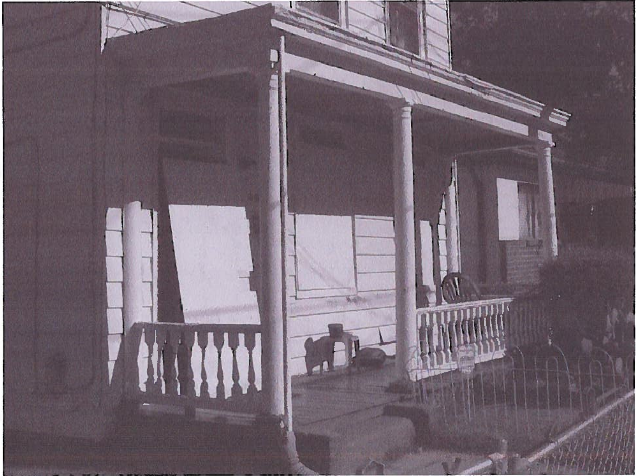
Detail of eastern elevation
