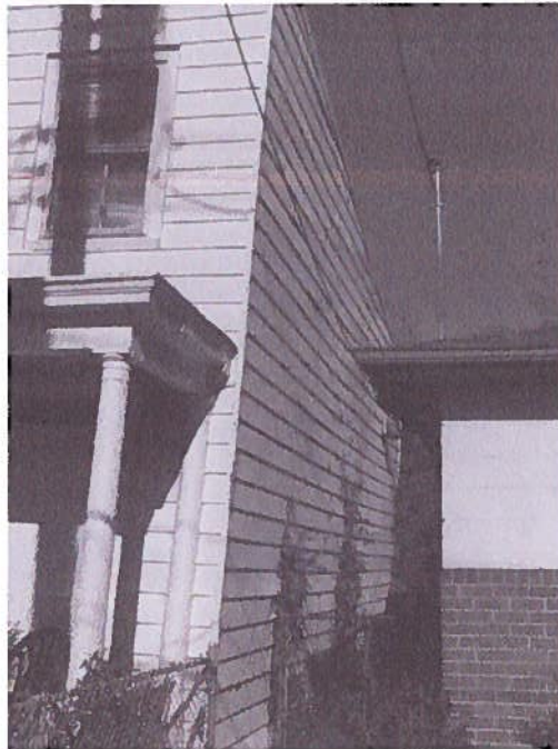
View of northern elevation from the east (taken from sidewalk)
