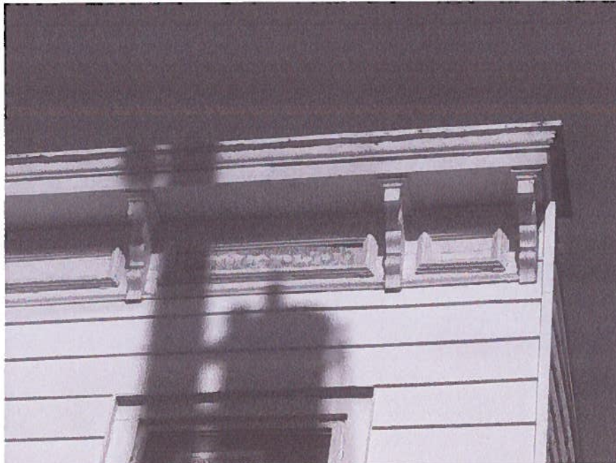
Detail of eastern elevation
