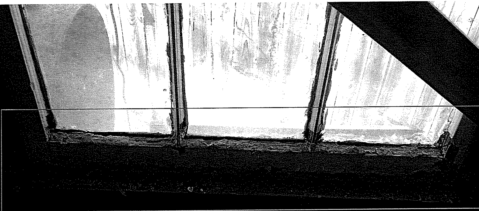
Downstairs Window No. 1 Bottom Sash Rotten Beyond Repair
