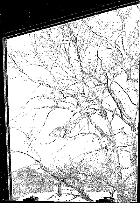
Upstairs Window -New Vinyl Window -Already Installed before Project Began
