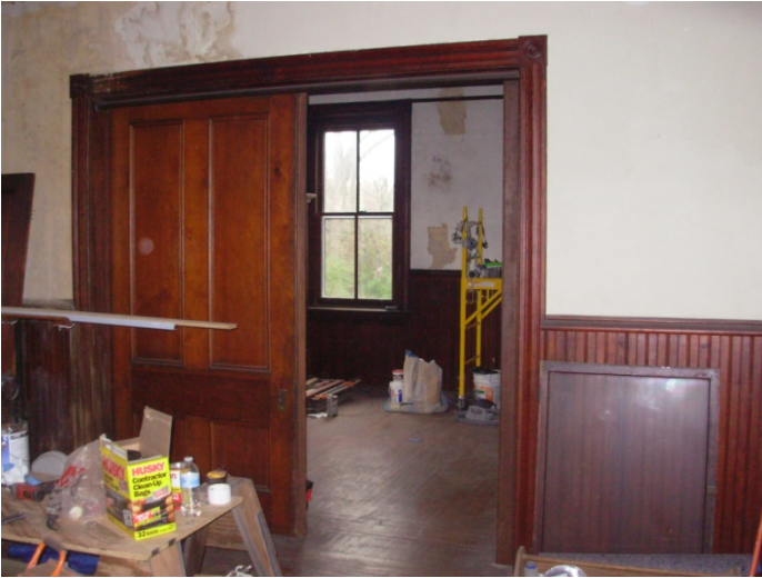
Existing pocket door between apartment unit and main house
