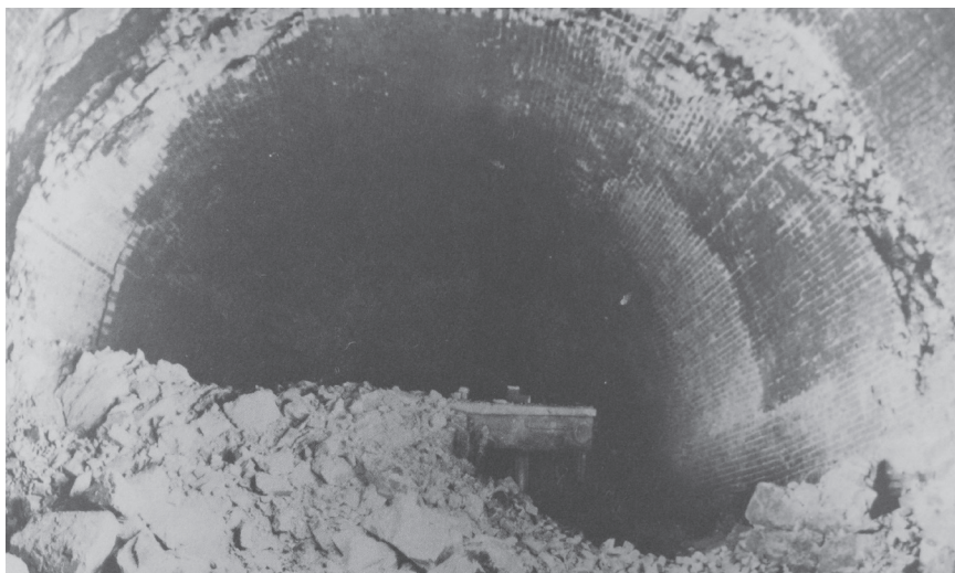
Section of Church Hill Tunnel. Locomotive Historical Society.
