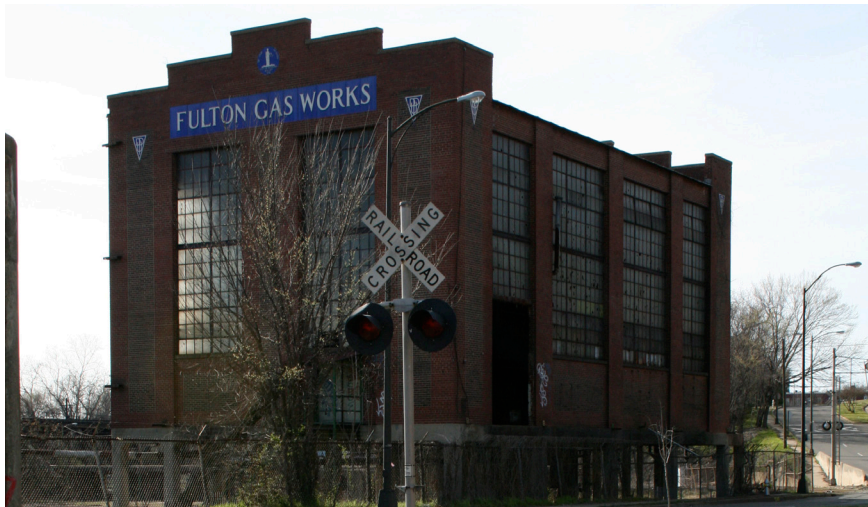
Boiler House from Williamsburg Avenue, 2011. Photo by Michelle Benoit.
