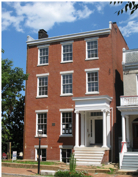
19 N 29th Street rear, 2010. Photo by Moseley Architects.
