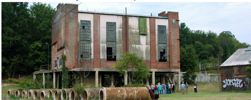
South View of Boiler House, 2010. Photo by Peter Sefton.
