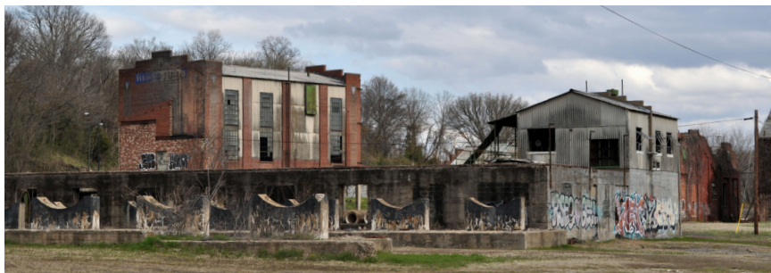
Reinforced concrete foundation of the 1908-1909 Retort House, 2011. Crystal Prigmore.
