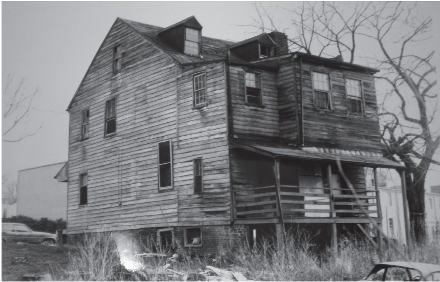
Back of the Woodward House, 1960's. Richmond Department of Housing.
