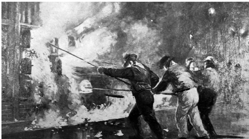
Employees stoking the fires of the retort house in the 19th century. 1936 Richmond Department of Public Utilities Annual Report.
