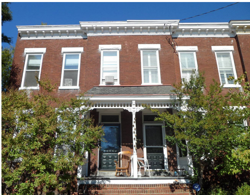
Row houses 2800-2806 which replaced the Carrington House, 2010. Photo by Kristin Rourke.
