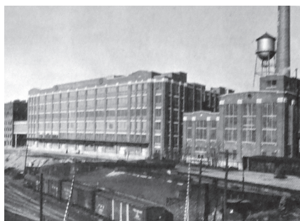
Exterior of Lucky Strike Building. Virginia Department of Historic Resources.
