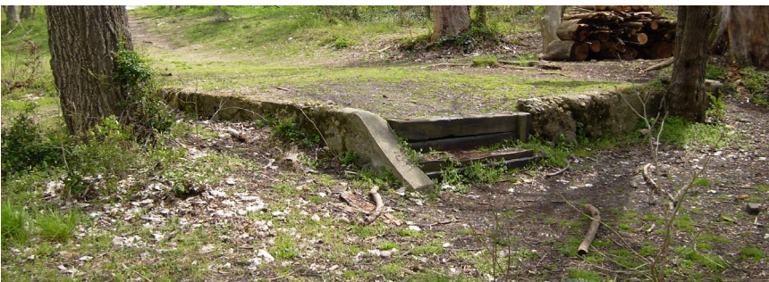
Foundation believed to be 615 State Street, 2011. Photo by Gray Graham.
