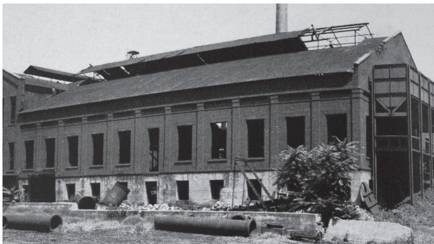
Shell of the 1908-1909 Retort House before demolition. 1939 Richmond Dept. of Public Utilities Annual Report.
