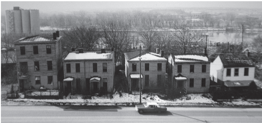
Williamsburg Avenue, 1960's. Richmond Department of Housing.
