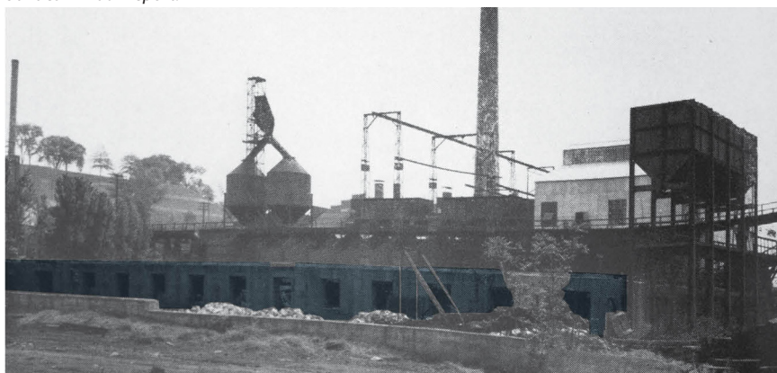
Reinforced concrete foundation of the 1908-1909 Retort House. 1939 Richmond Dept of Public Utilities Annual Report.
