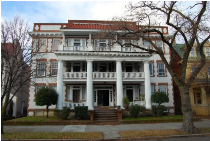
110 North Boulevard (The Belmont)
