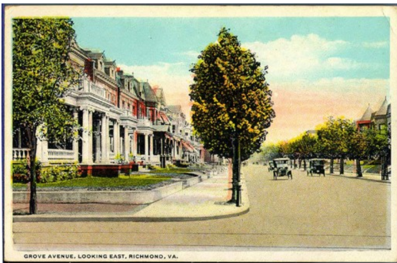
Grove Avenue looking east (undated)
