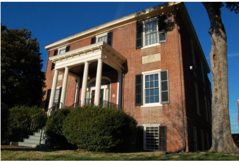
1142 West Grace Street (Columbia House 1817/1818)
