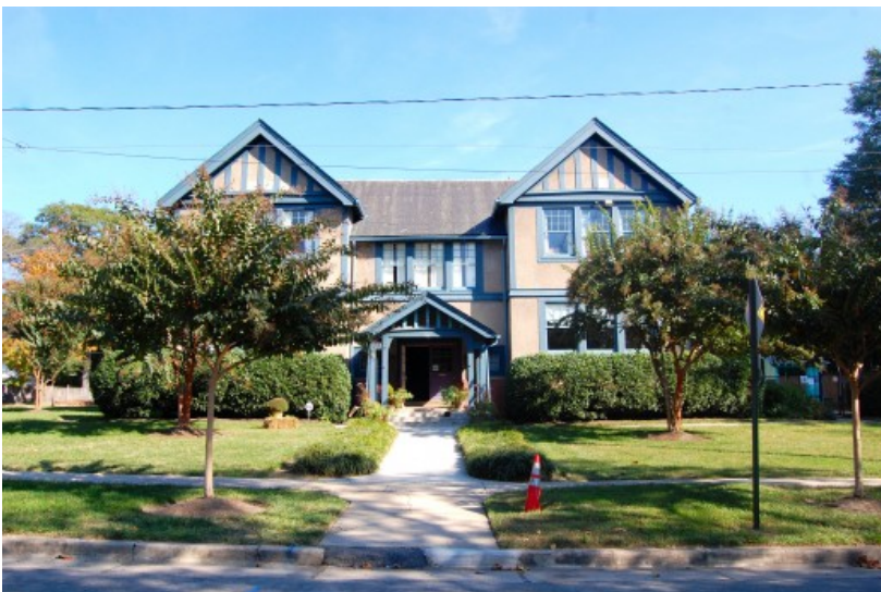
Lewis Ginter Community Center (3421 Hawthorne Avenue)
