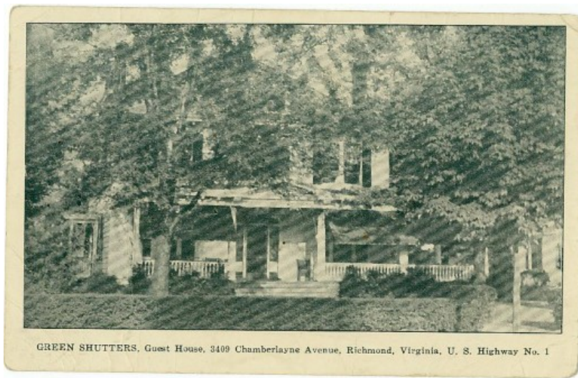
3409 Chamberlayne Avenue (from Chamberlayne Avenue)
