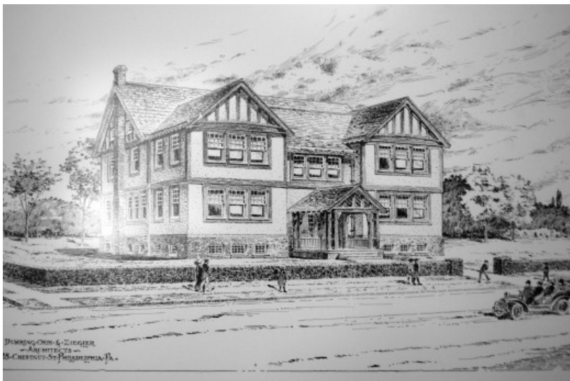
Lewis Ginter Community Center (3421 Hawthorne Avenue)
