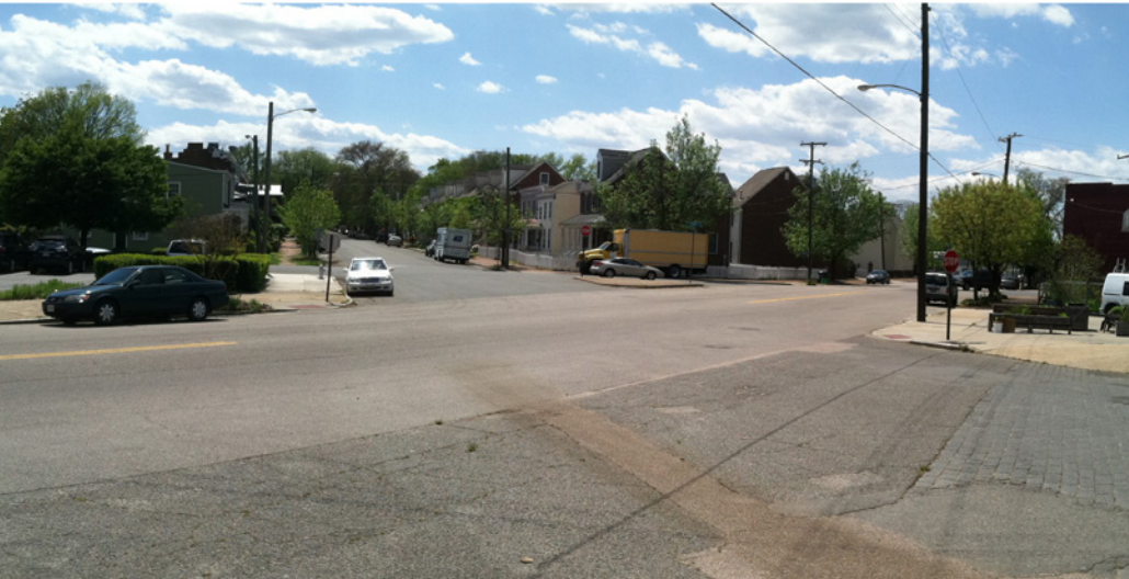
EXISTING CONDITIONS LOOKING SOUTHWEST
