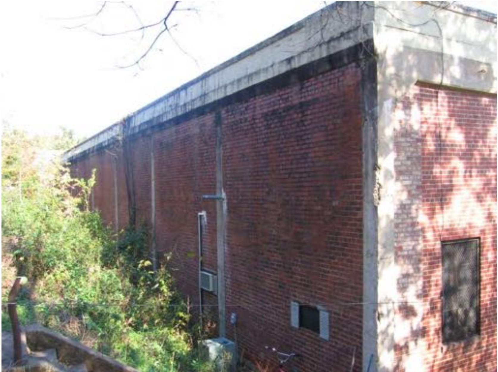
SW Corner. looking NE
