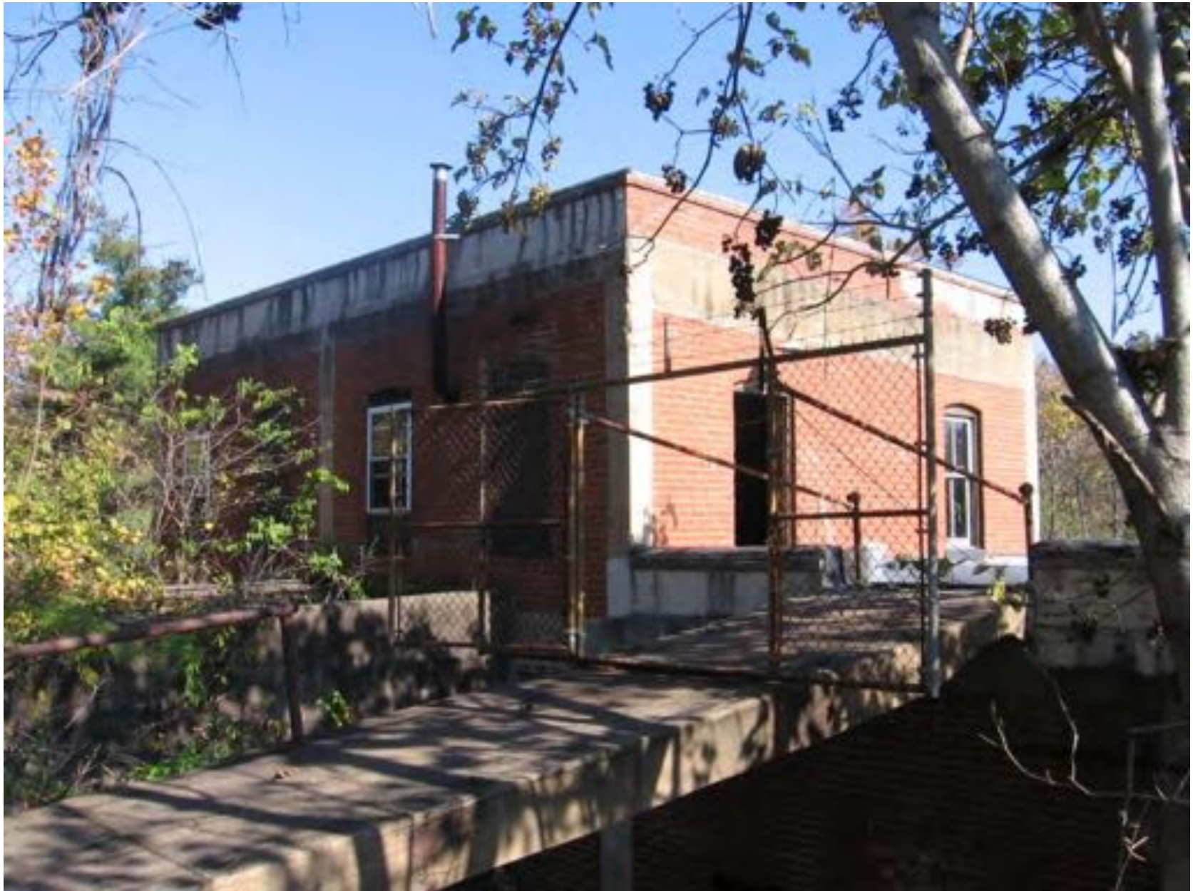
Walkway from trolley track to Office on roof, looking NE
