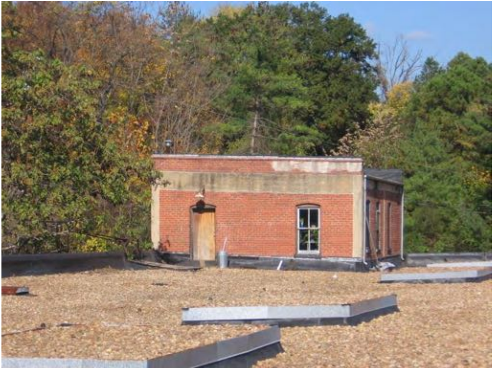
Roof, looking NW
