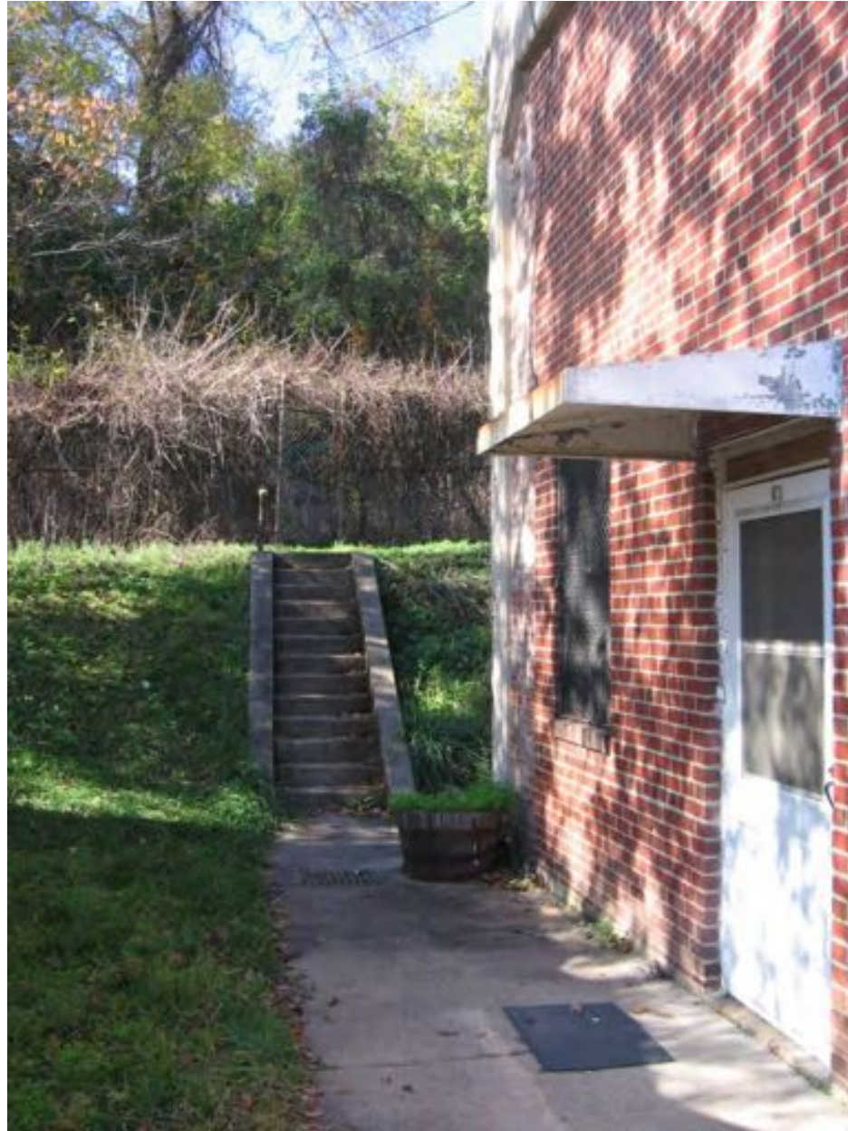
Stair to trolley track, looking W
