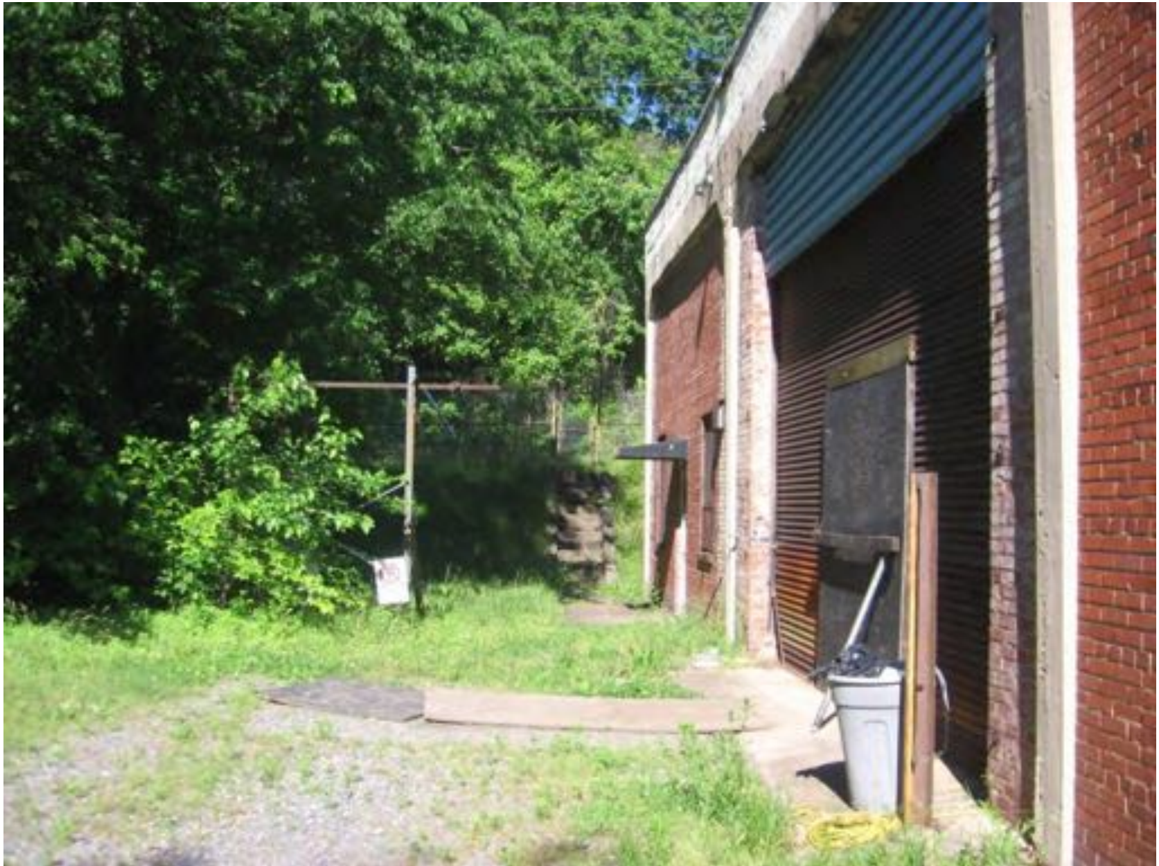
South Elevation, stairs to trolley line, looking NW
