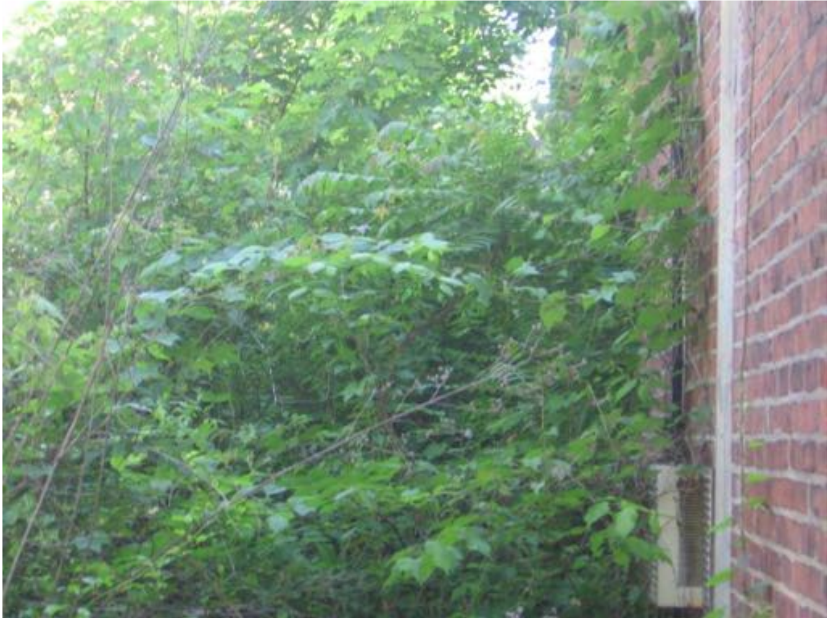
West Elevation, looking NE
