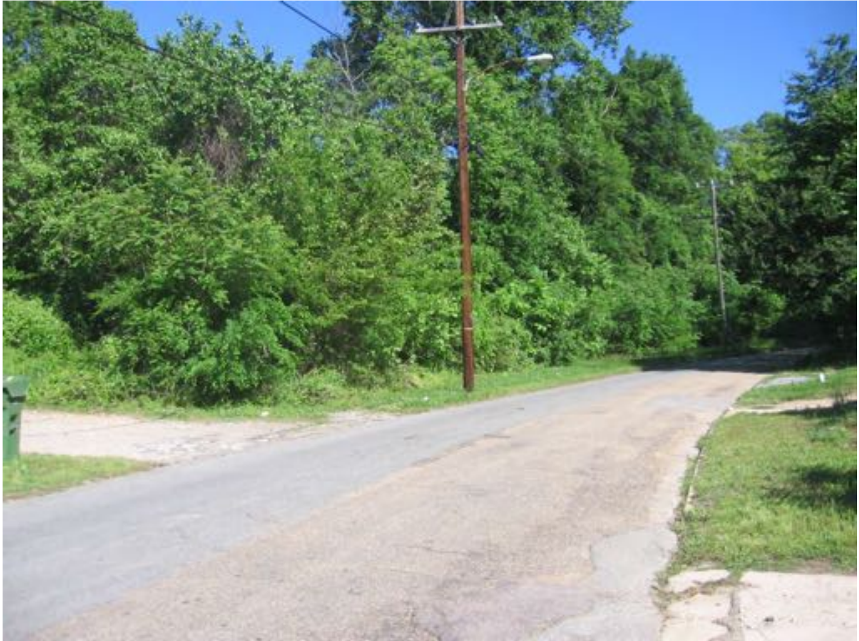
Glenwood Avenue looking NW
