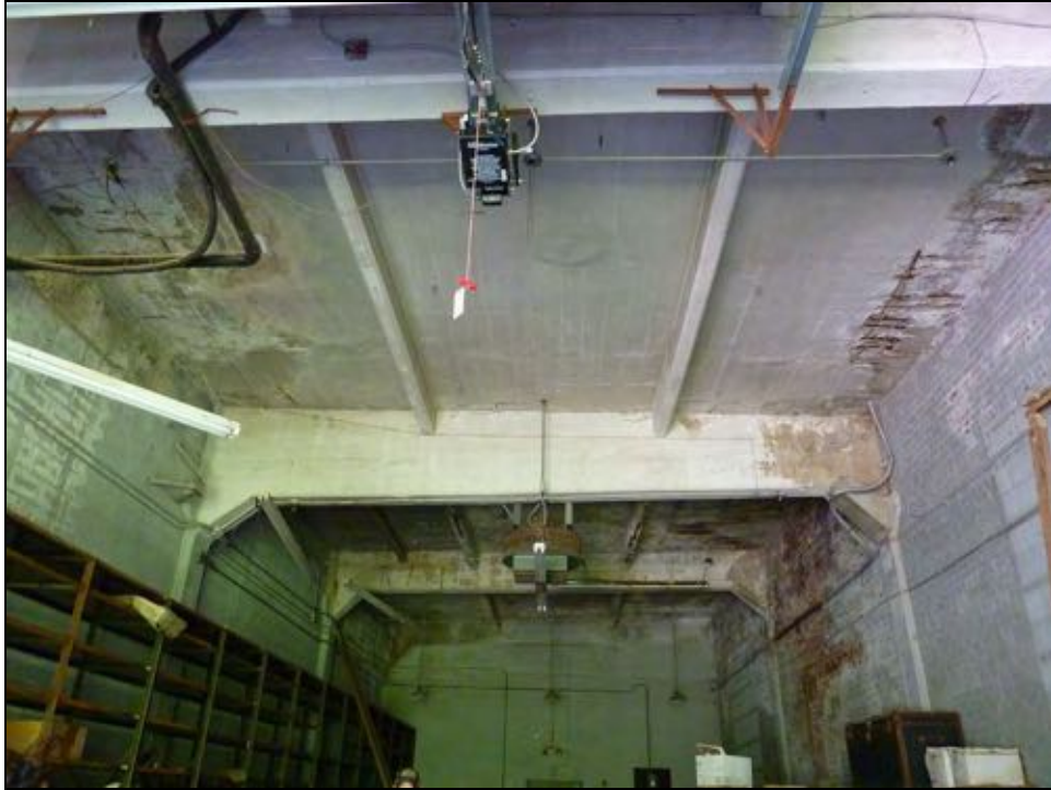
Figure 5-18: Exposed concrete structural elements, facing south
