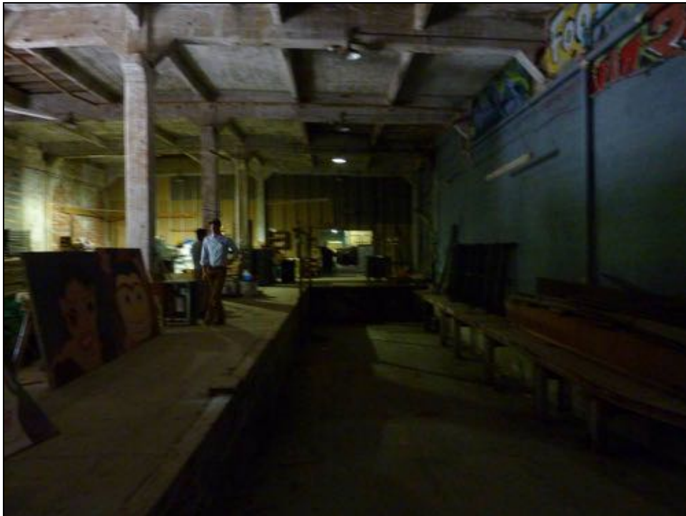
Figure 5-19: Depressed ramp and service area, facing south
