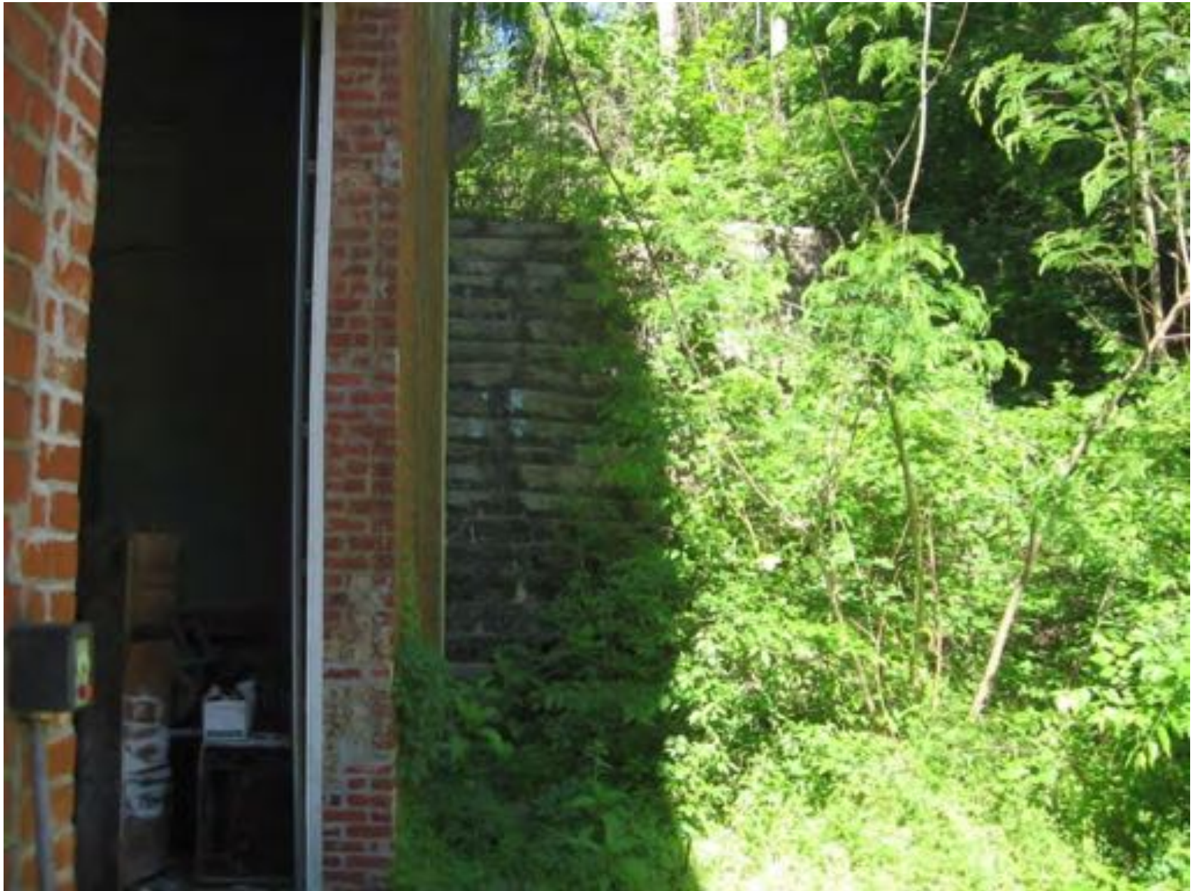
Retaining Wall at NW corner, looking W
