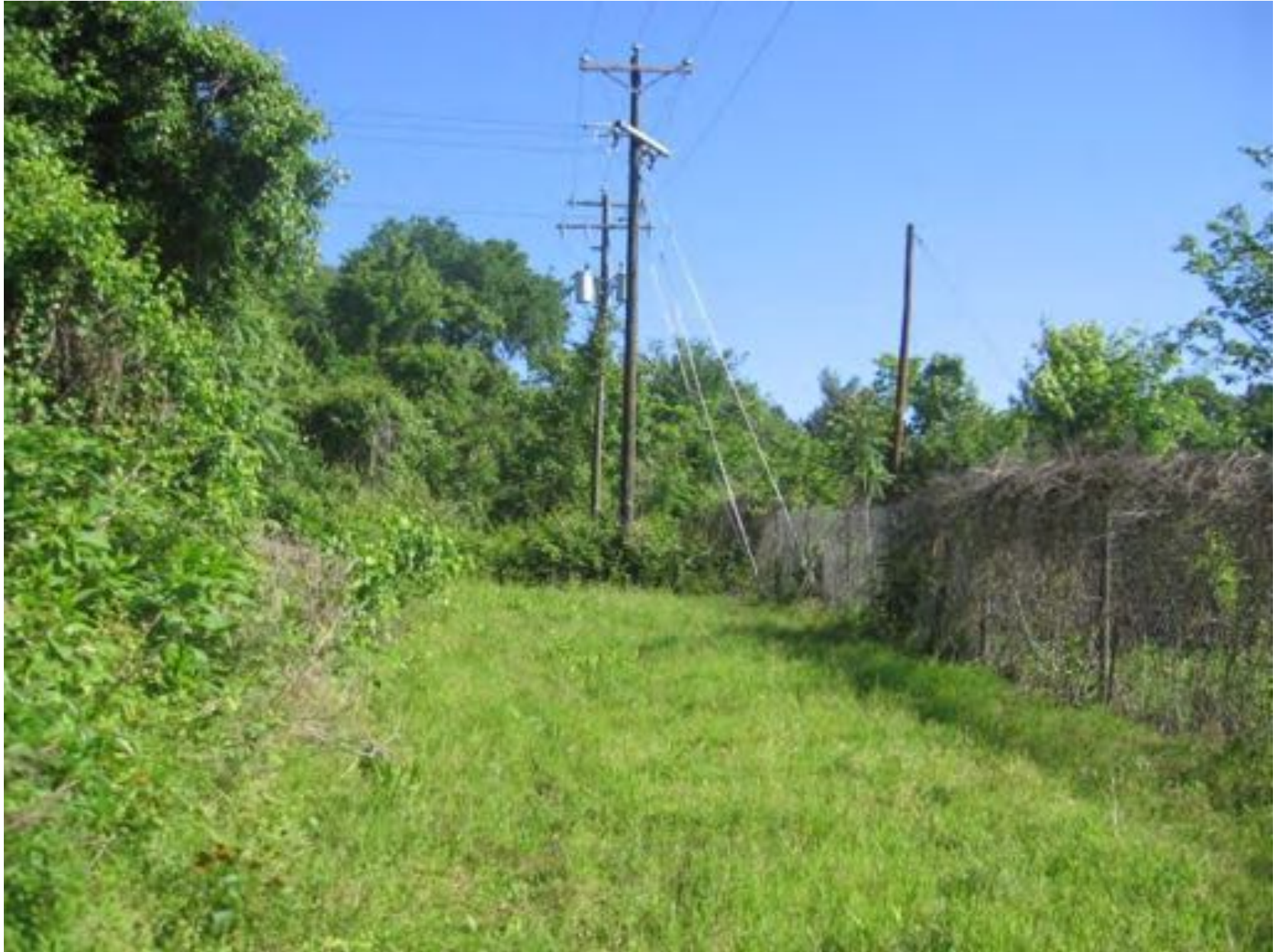
Location of trolley line (embankment to west of building) looking N
