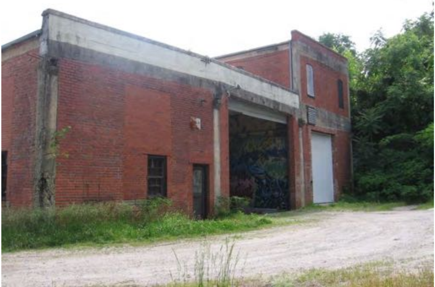
North Elevation, looking SW
