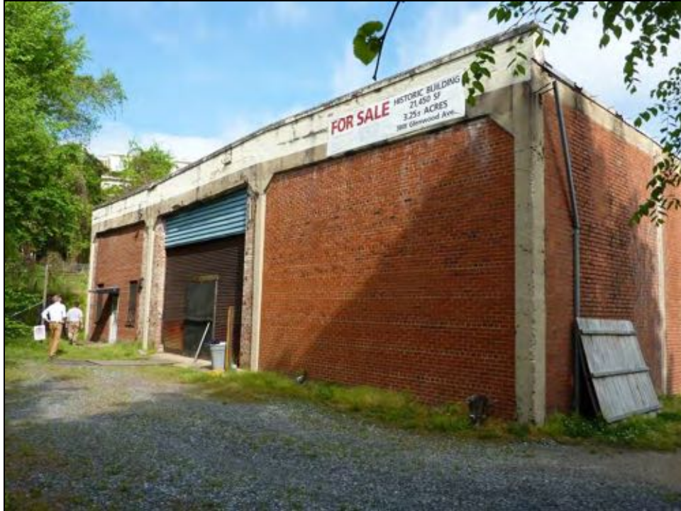
Figure 5-12: View of three-bay front (south) end, facing northwest
