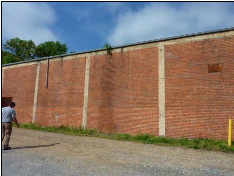
Figure 5-11: Concrete frame structural system with brick curtain walls on east side of building, facing west
