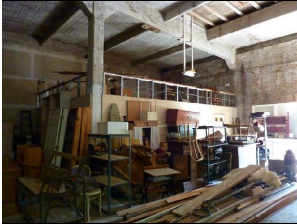
Figure 5-17: Partitioned area at northeast corner of building, facing northeast
