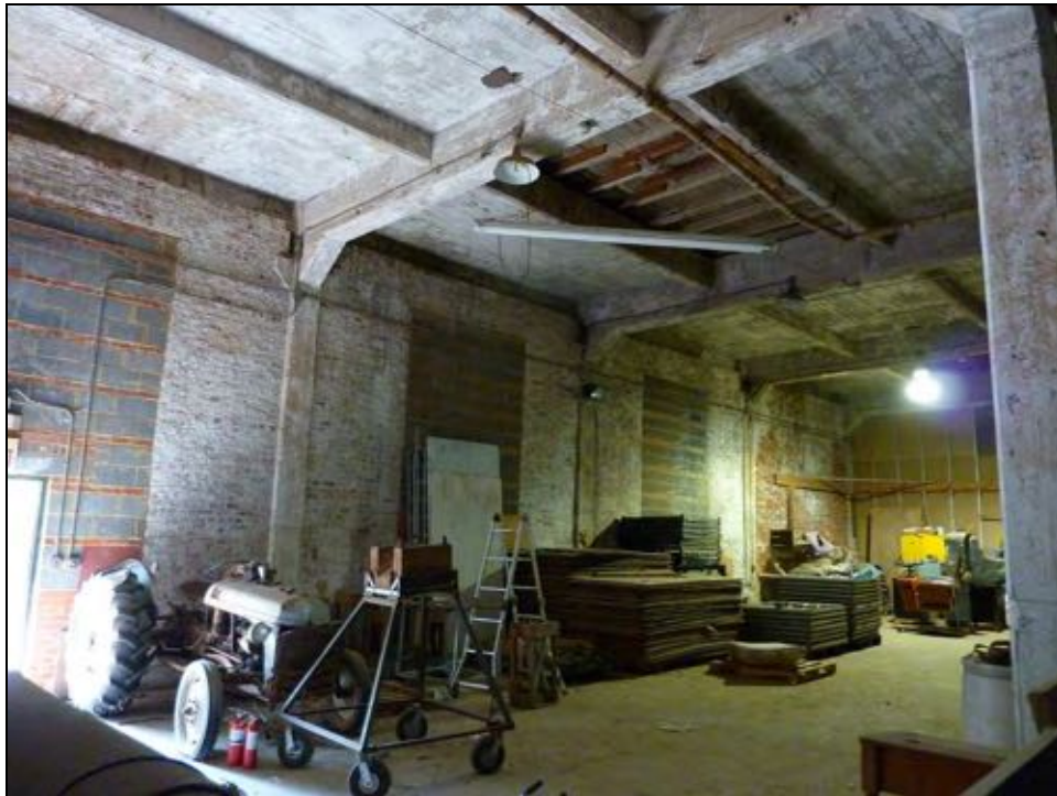
Figure 5-21: Infilled windows and skylights, facing southeast
