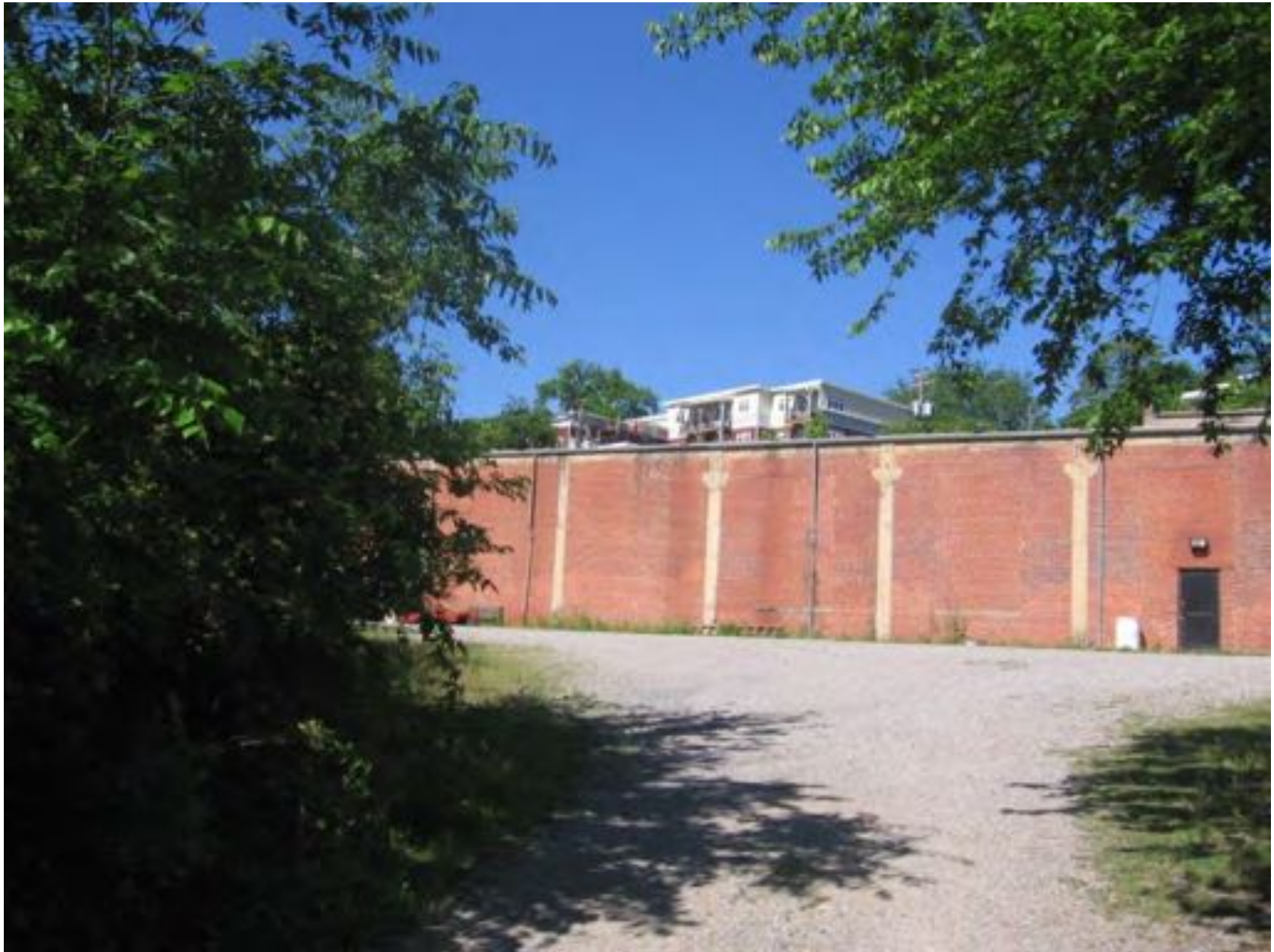
East Elevation, new construction at top of hill beyond, looking SW
