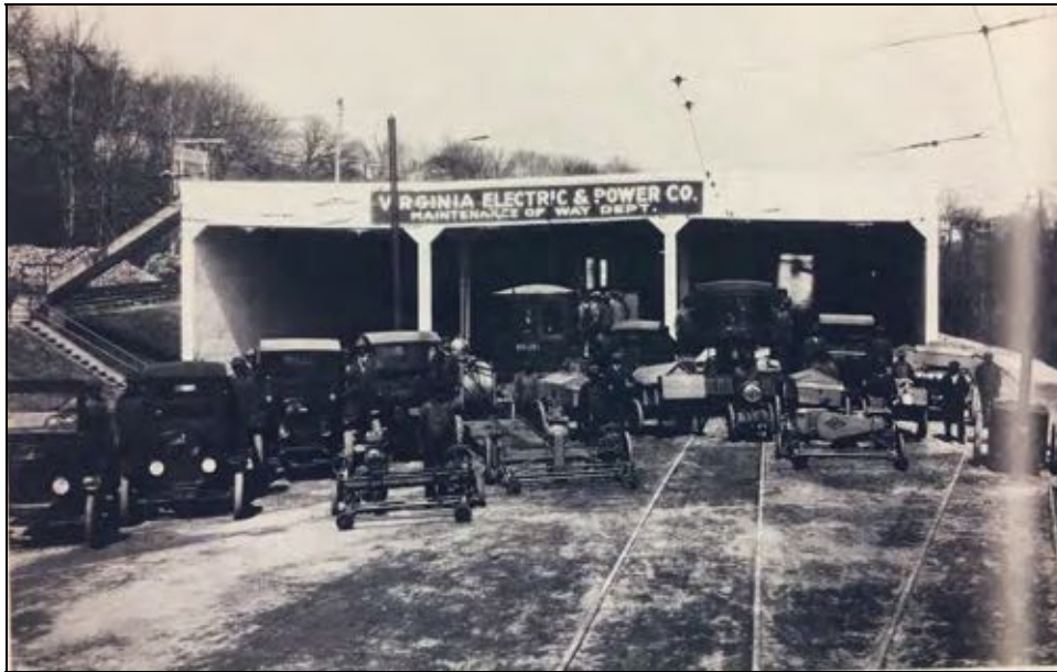
Figure 5-22: View of car barn building, circa 1925, facing north. Source: VDHR
