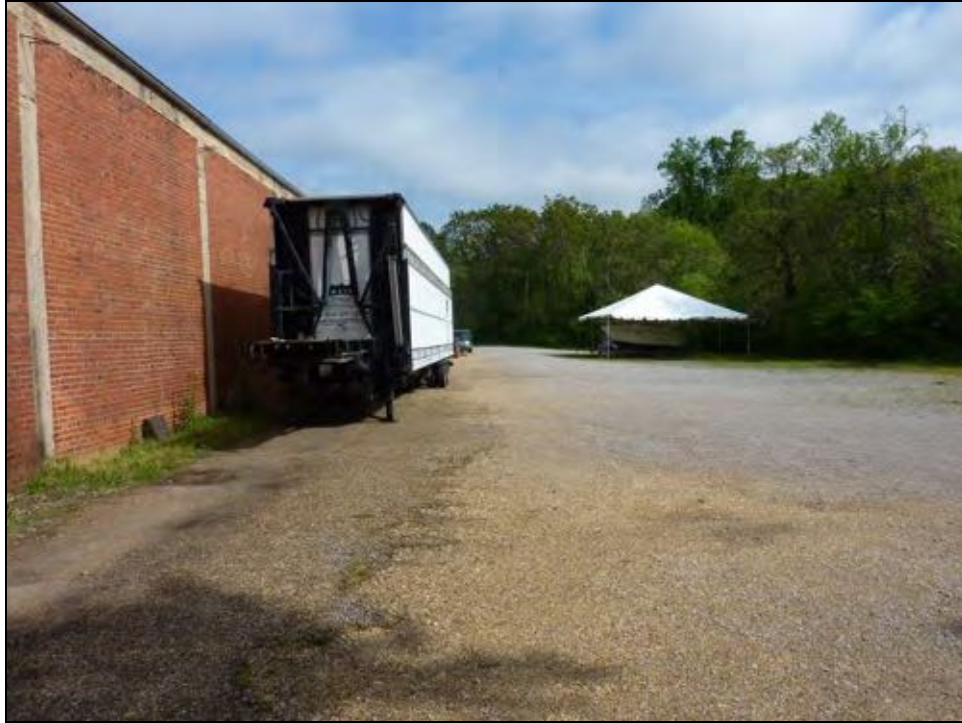
Figure 5-7: View of parking lot along east side of building, facing north
