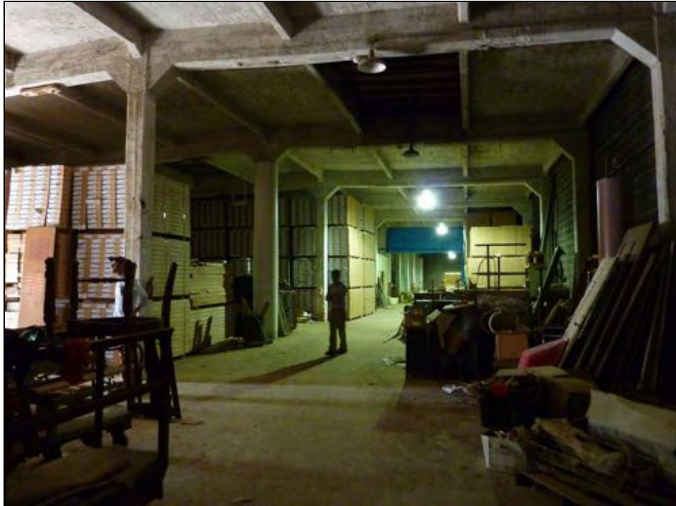
Figure 5-16: Interior space with concrete post bay divisions, facing north
